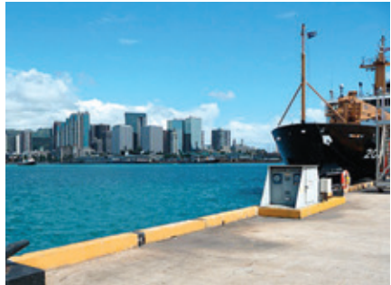
View of Downtown from the Coast Guard pier.
